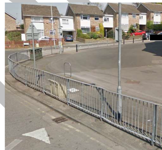
11. Long guardrail here adds to the overall street clutter (Delta Gain, Carpenders Park).
