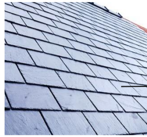
Grey slate roofing
