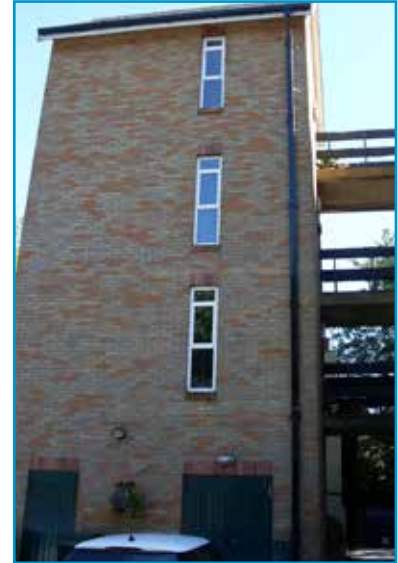
Stair tower serving the former mill
