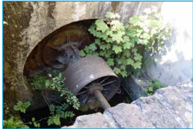
Turbine remains in a wheel house
