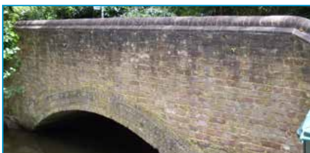
Road Bridge over River Gade
