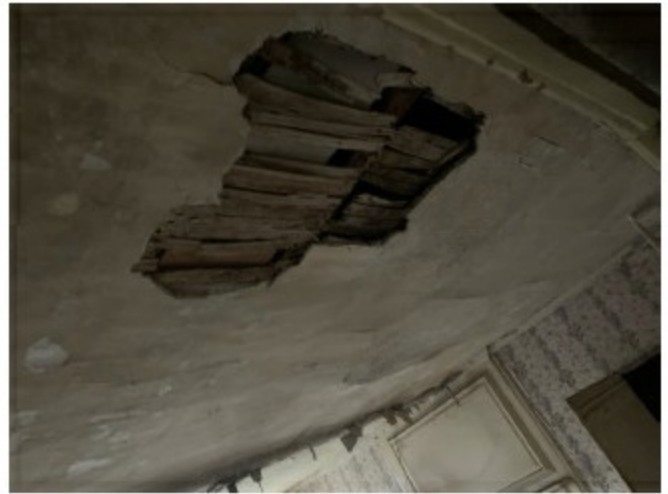
First floor ceilings proposed to be removed for investigatory works/ repairs to timber floors
