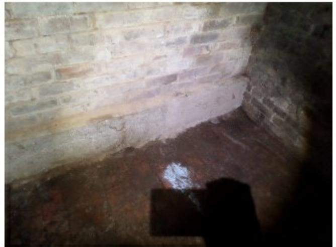
Brick Cellar floors – Higher level at foot of stairs & lower level below kitchen with concrete plinth
