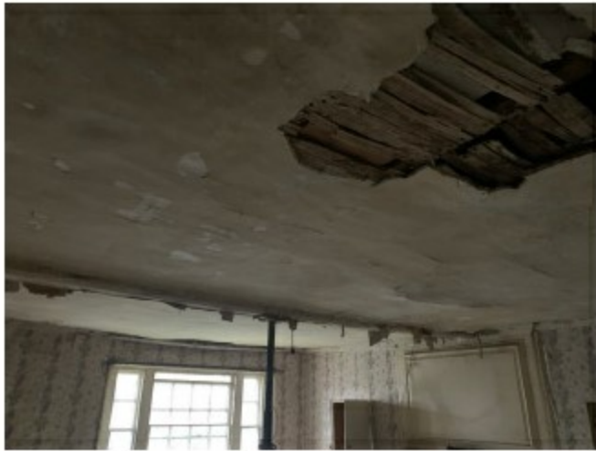
First floor ceilings proposed to be removed for investigatory works/ repairs to timber floors
