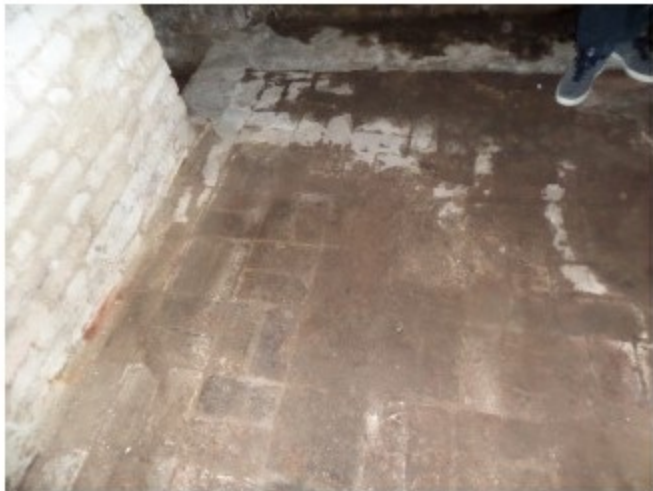
Brick Cellar floors – Higher level at foot of stairs & lower level below kitchen with concrete plinth
