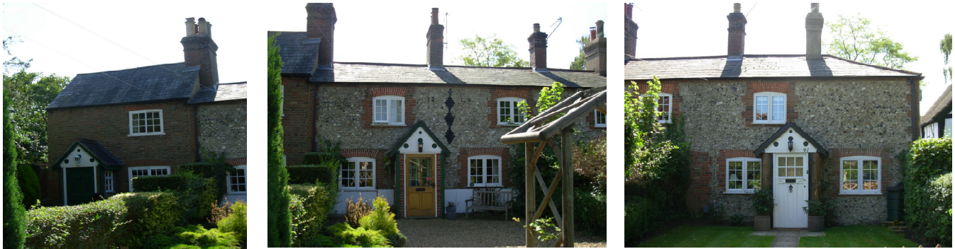
Figures 34, 35 and 36: No. 93, 95 and 97 Kitters Green - Locally listed
