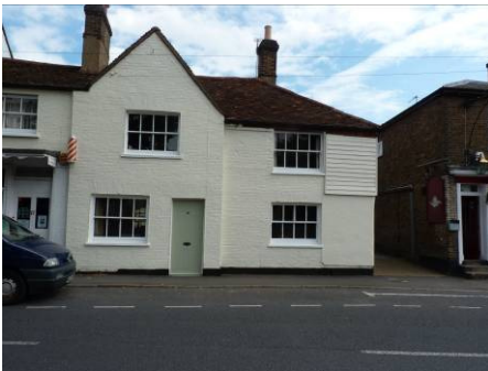
Figure 14: No 17 High Street.
