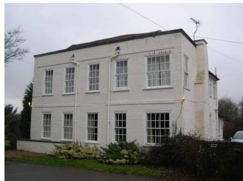
Figure 10: The Vicarage—Grade II Listed
