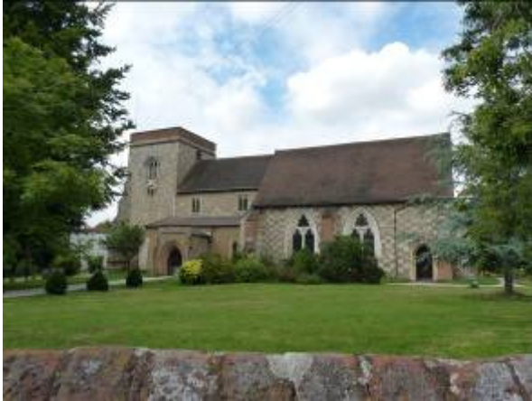
Figure 5: Church of St Lawrence—Grade I Listed Building
