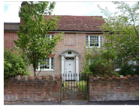
Figure 15: No 25 High Street.
