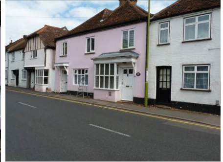
Figure 13: No 7, 9, 9a and 11 High Street
