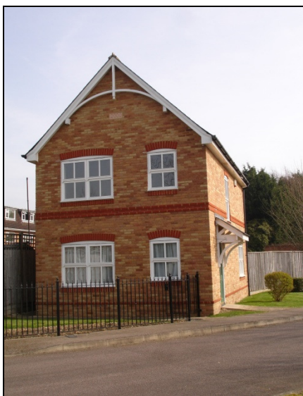
Figure 28 - No. 1 Cherry Croft, looking East.
