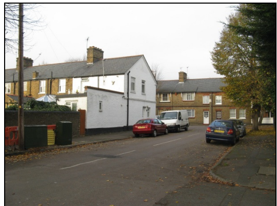
Figure 22 - A view from further up the South access road, looking towards the smaller terraced houses on the North side.
