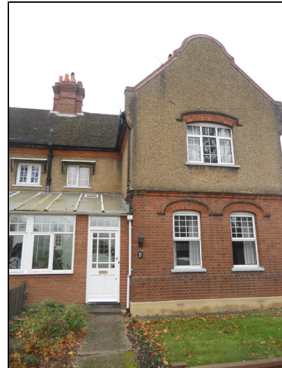
Figure 33 - No. 4 Dickinson Avenue, with Dutch gables in contrast to the other buildings within the Area.
