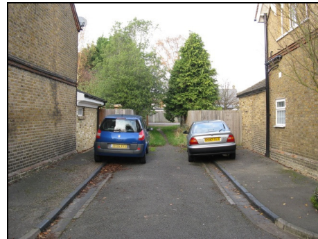
Figure 6 - One section retains earlier black kerb stones and road surface material.
