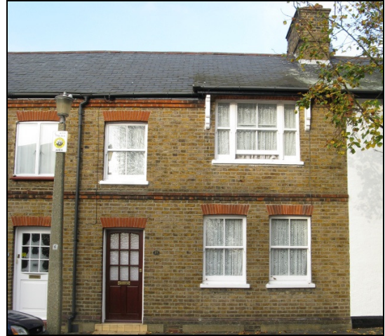
Figure 31 - The smaller terraces are also adorned with attractive, but more subtle, decorative brick moulded string courses and window arches. Together with the attractive sash windows, these form a neat façade.
