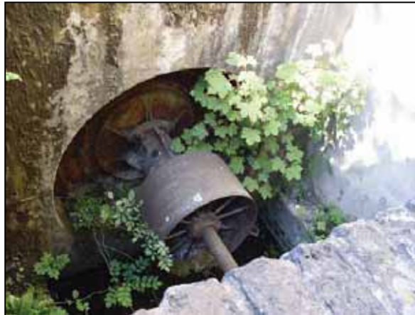
Turbine remains in a wheel house
