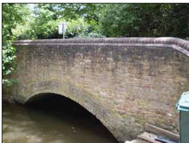
Road Bridge over River Gade
