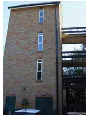
Stair tower serving the former mill
