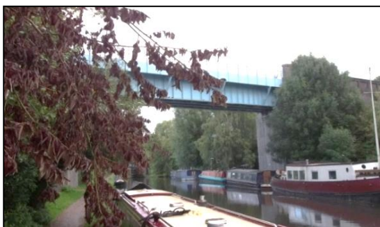
Cr Railway bridges (this one at Cassiobridge) 7] [re
