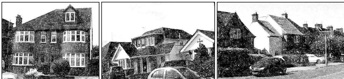
Illustrative examples of unsympathetic extensions (a) asymmetric modifications, (b) bulbous protrusion of roof, (c) inharmonious materials
