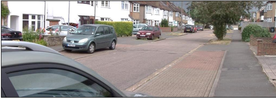
Parking hard shoulders at Bateman Road
