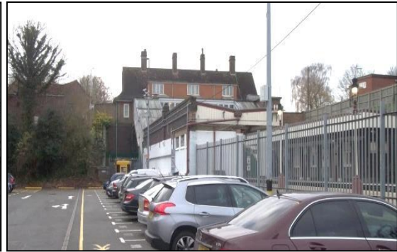
(b) car park and platform buildings
