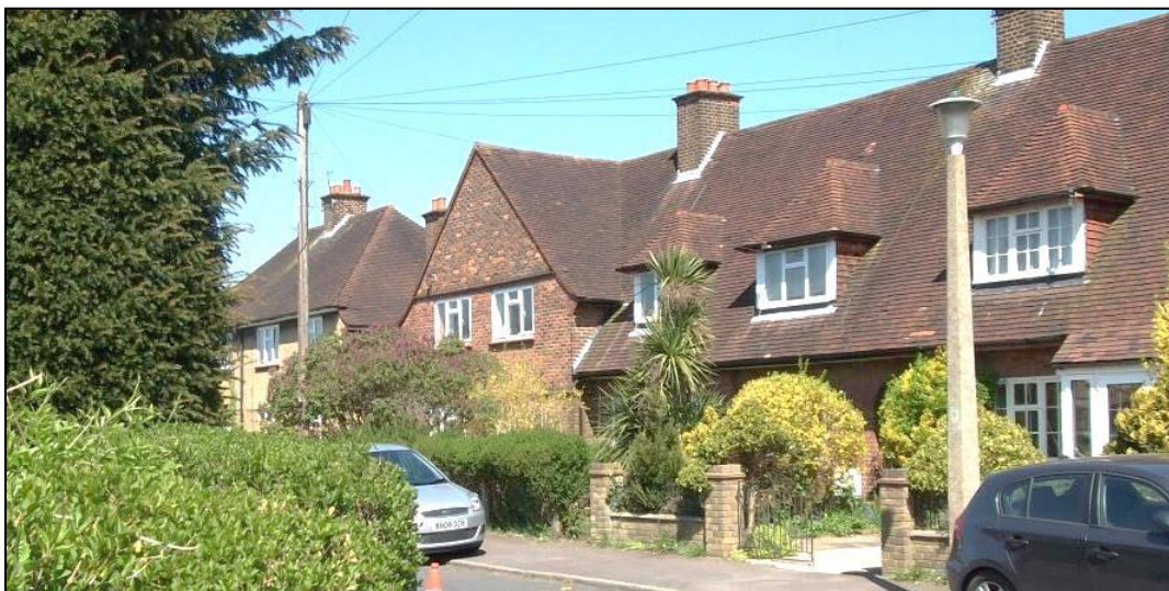
Gonville Avenue - original council housing dating from 1921
