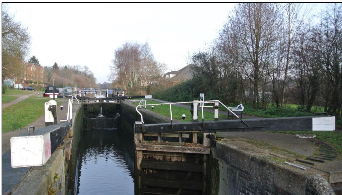
The Canal in Character Area 11 (Common Moor Lock)
