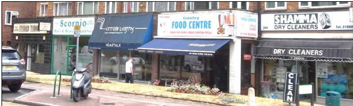
Shopping parade on Watford Road showing discordant shop front design
