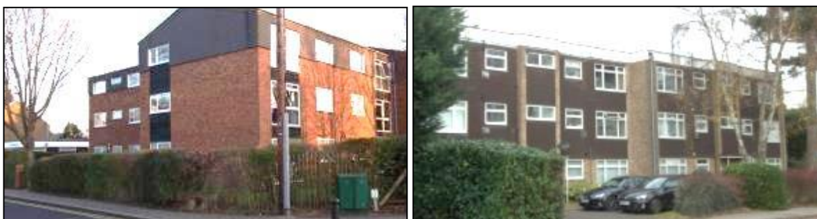
Left: The utilitarian Guildhouse flats built in the 1960s on the site of the former meeting hall – the tree on the left is the largest remaining on New Road. Right: very Spartan 1960s flats close to Croxley Station
