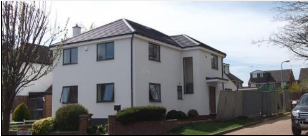
Imposing and well-proportioned reconstructed house (formerly an isolated bungalow) on corner site at 31 Rochester Way which “fits” the “urban grain” in scale but the roof has a different colour and texture
