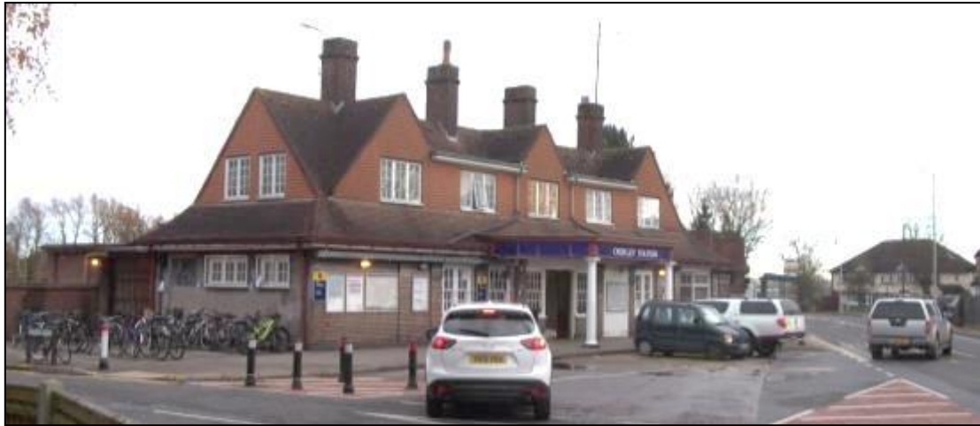
Croxley Station opened in 1925, still largely in its original condition
