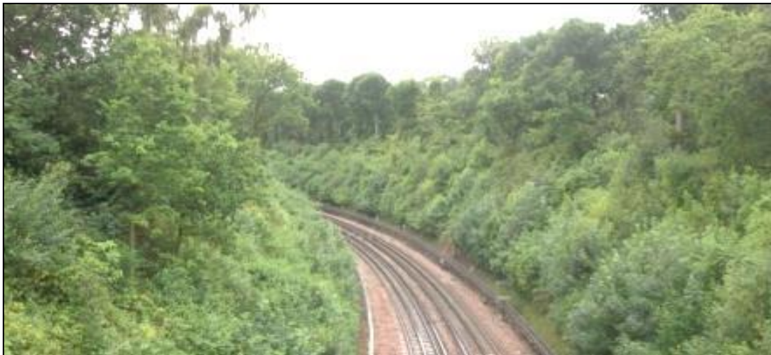
The Metropolitan Railway cutting looking west from Harvey Road Bridge
