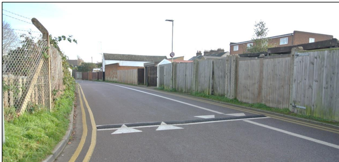
Community Way (showing the shared surface footway marking and speed control ridges)
