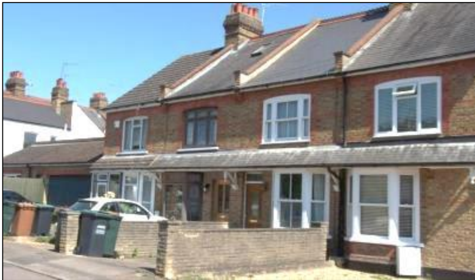
Paved forecourts and miscellaneous designs of replacement windows detract from the unity of a late Victorian terrace in Yorke Road
