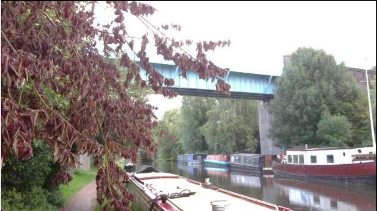
Metropolitan Line Railway Bridge over the Grand Union Canal at Two Bridges
