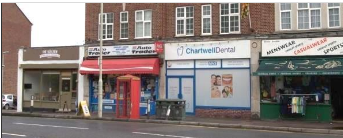
Better alignment and more discrete signage design in the older parade in Watford Road near Croxley Station
