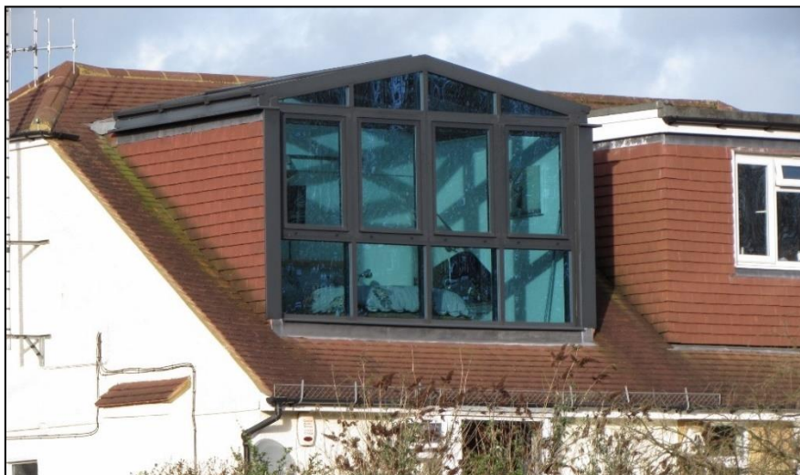
Dormer facing allotments at rear of Frankland Road property
