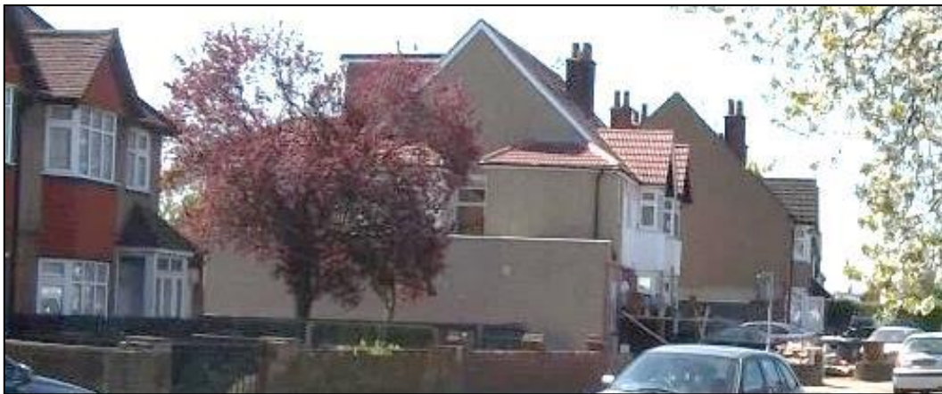
“Ungainly overdevelopment” of extension to Edwardian house in Watford Road
