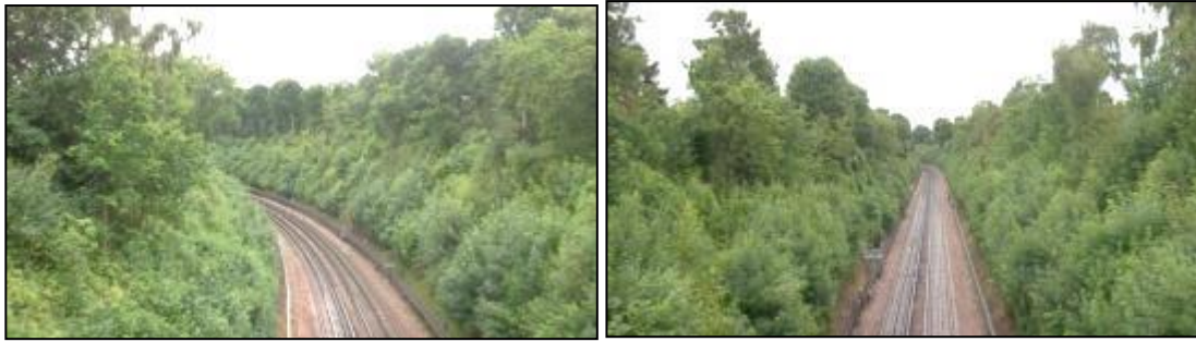
View of cutting from Harvey Road Bridge looking (a) west and (b) east
