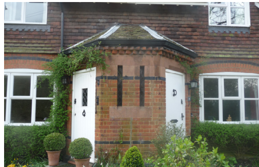
Front elevation of Bacher (l) and Worth (r) Cottages with a unique character of the Conservation Area
