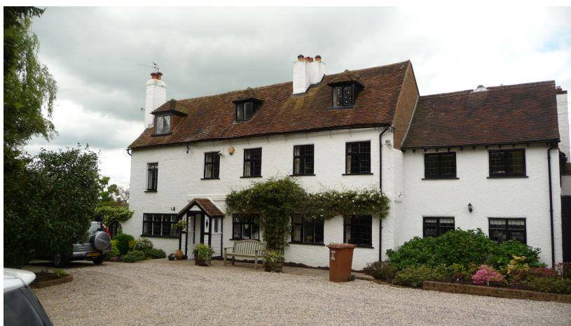
Batchworth (left) and Ebury Cottages
