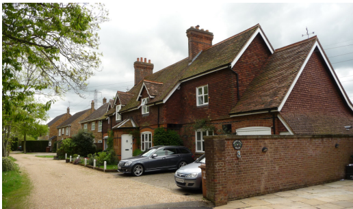
White Hill, Worth & Bacher Cottages looking east
