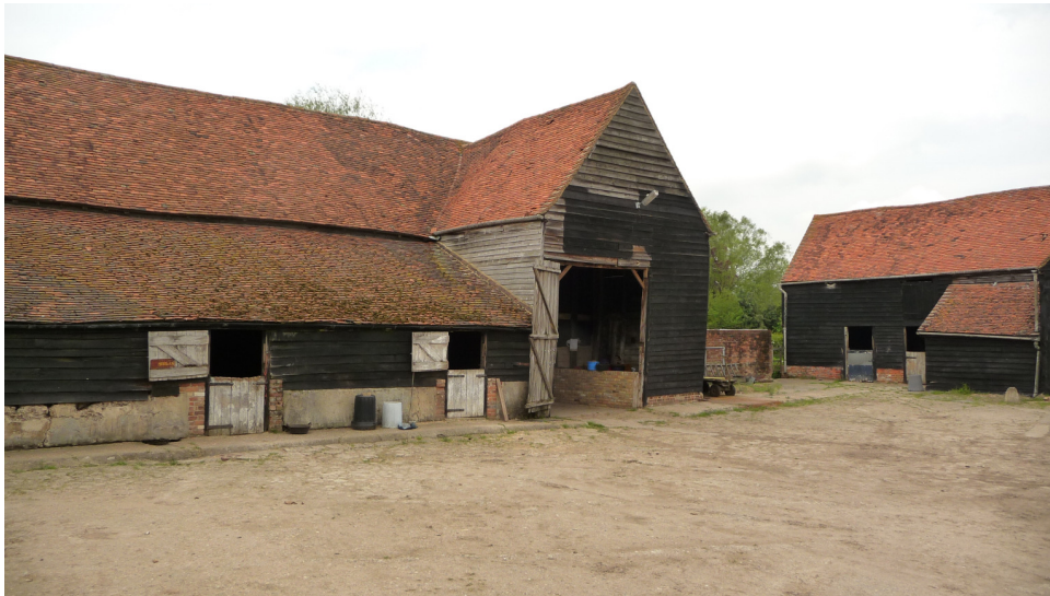
The barn situated 25m north west of the farmhouse
