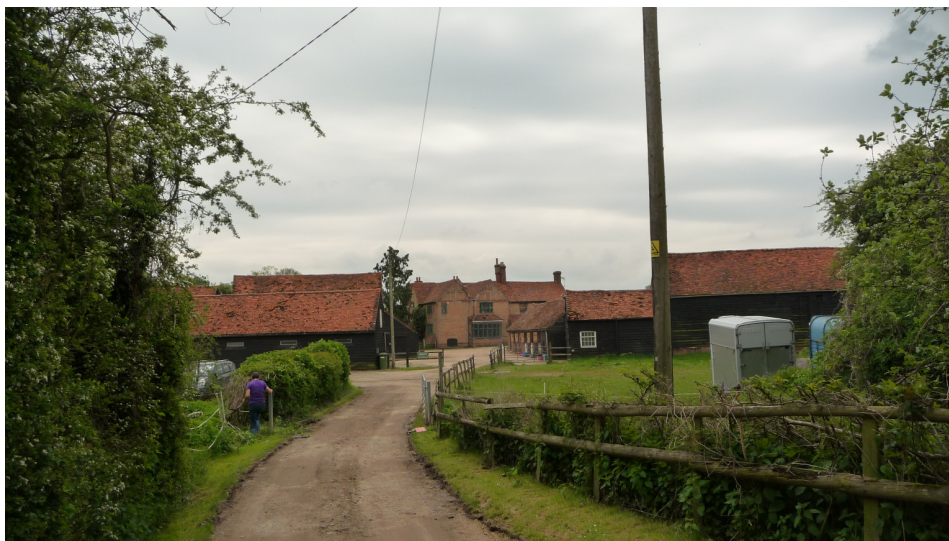
Looking south from the canal bridge, views of the Farm House are gained from between the associated barns
