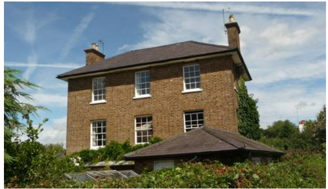
The southwest elevation of Stocker's House
