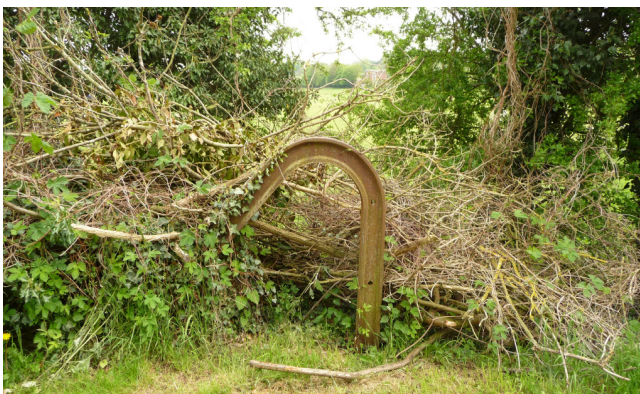
There are many anti-tank obstacles across the Grade II Listed bridge
