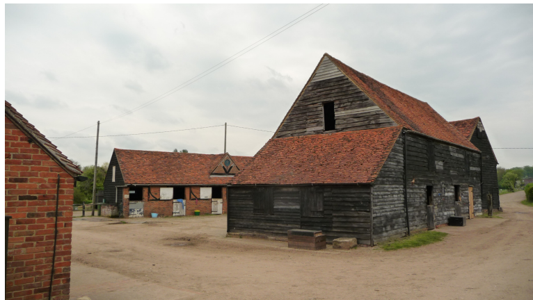
The two barns 20m North East of the farmhouse
