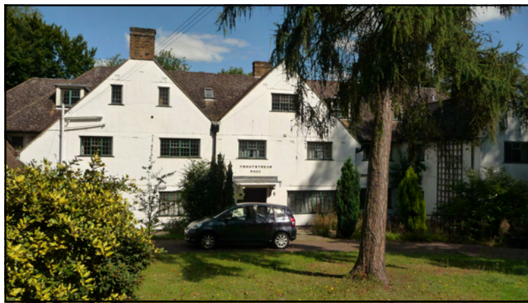
South west elevation of Troutstream Hall
