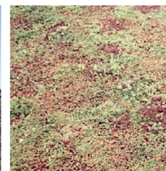
Sedum Roof Covering
