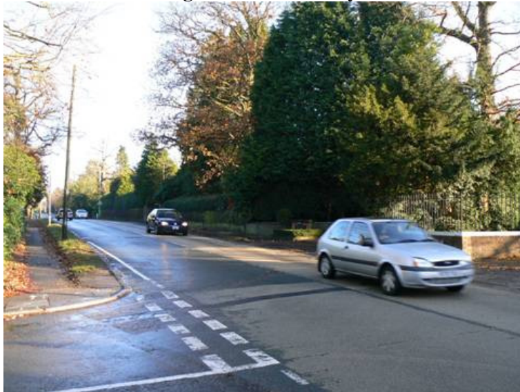
Looking north up Watford Road
