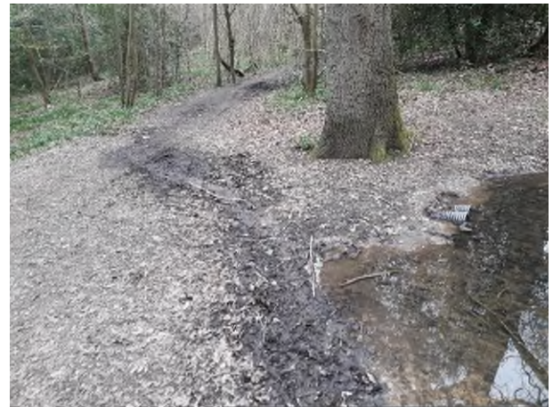
Pond overflowing across path
