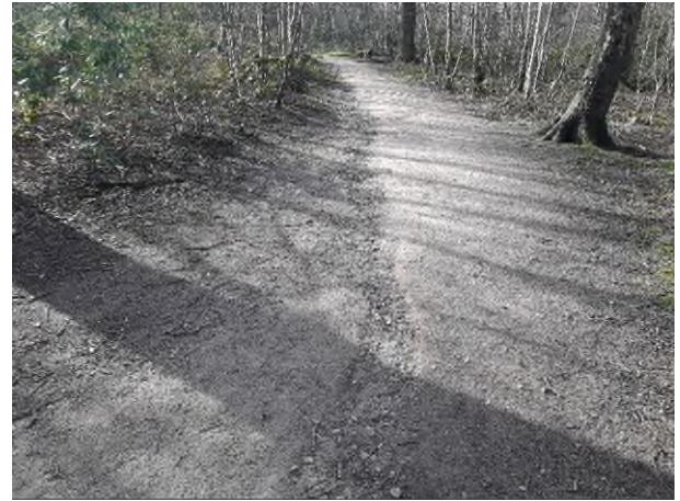
Channelling to path surface
