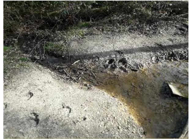
Erosion of lower bank
