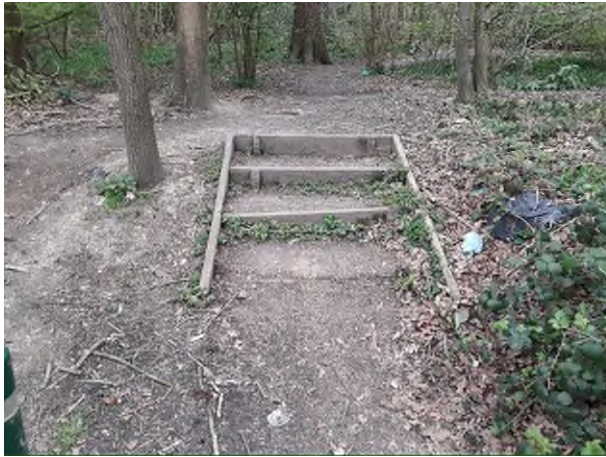
Steps for refurbishment
